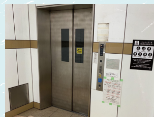
Wheelchair Accessible Elevator
